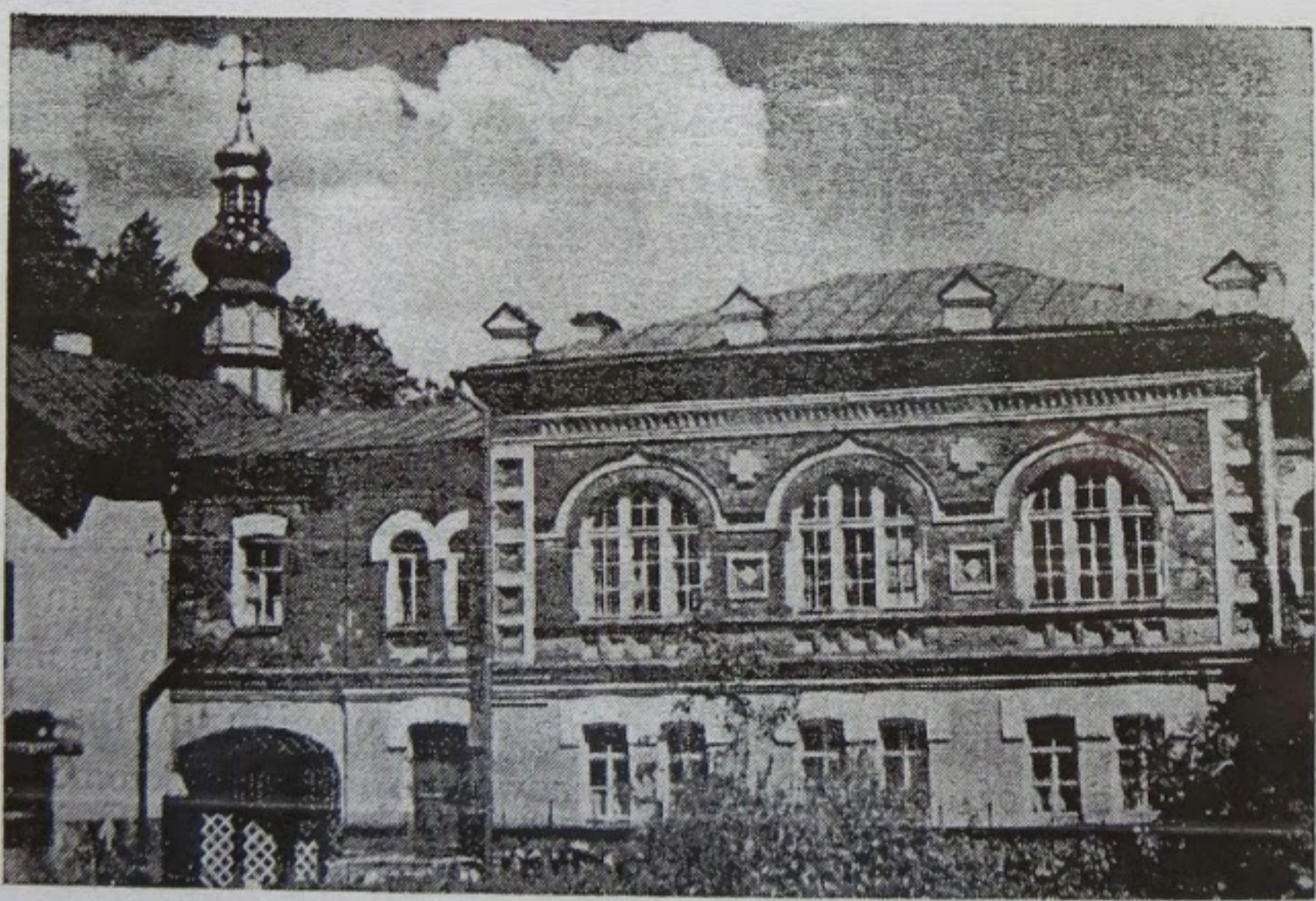
Pskov-Caves Monastery: St. Lazarus church with adjacent Refectory building where Schema-Bishop Macarius was killed in one of the ground-floor cells
